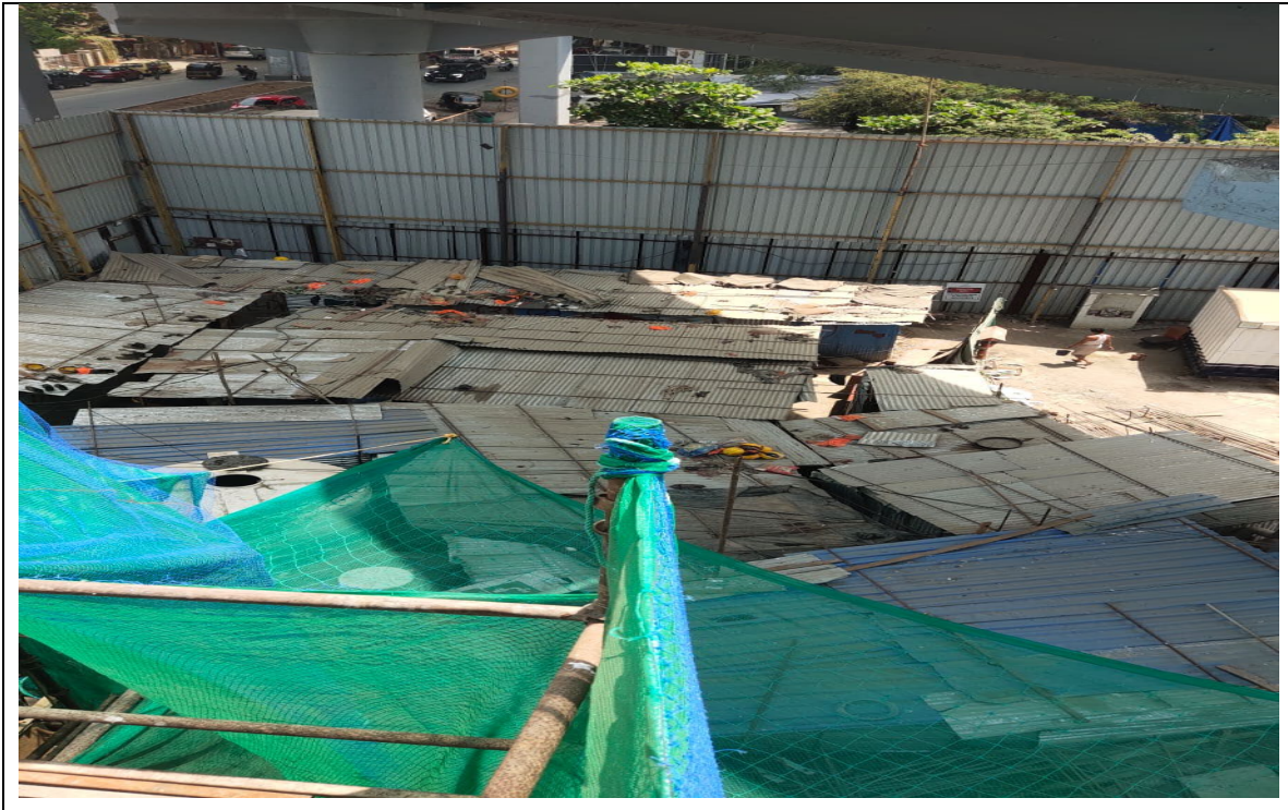
Labor camp top view with their safety inspection as per scheduled.
